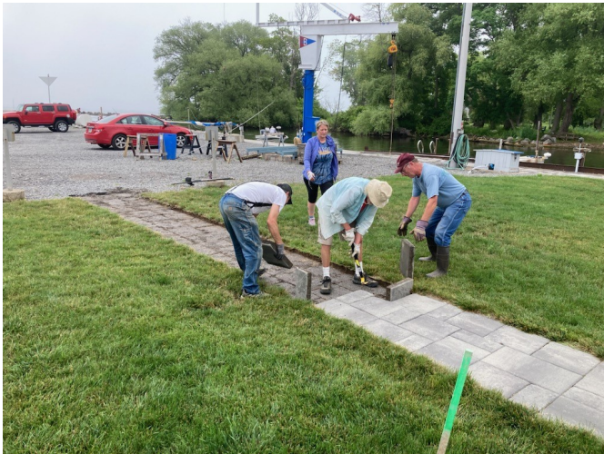
Moving pavers in advance of sewer work.
