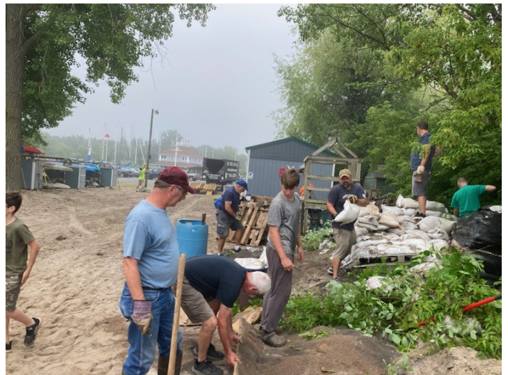
Disposing of the old sandbags.
