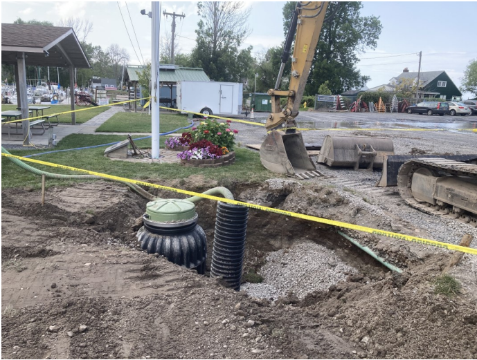
The new grinder was installed at the club this week for the sewers. Photo credit: Rich Wiest
