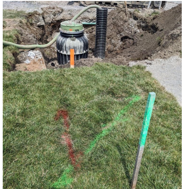
Looking north: Elect. conduit (red), line to pump-out shed at creek (green) & perforated
