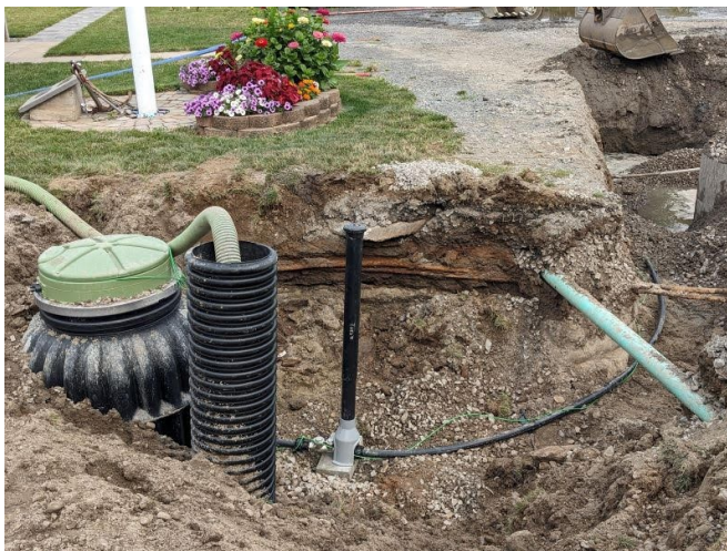
Looking west: Dewatering, new shut-off valve, & lots of existing utilities.
