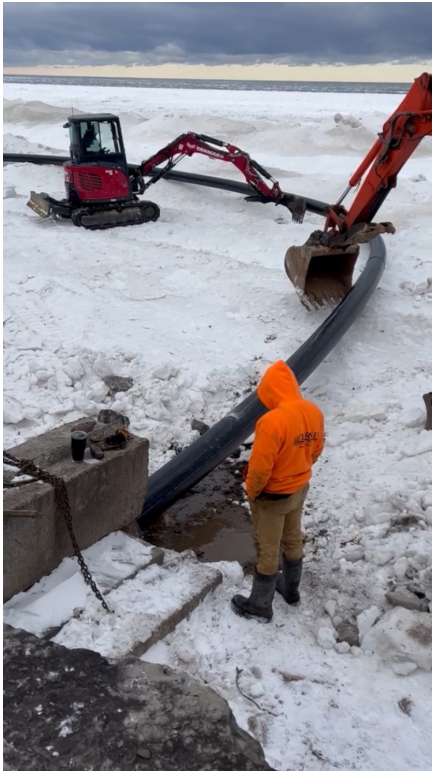
Some things can only be done along the lake in the winter. Town of Hamlin feeding a new 300 ft drainage pipe thru an existing damaged conduit off Westphal and Sandy Shore Drive the week of January 13. Submitted by Jeff Spring.
